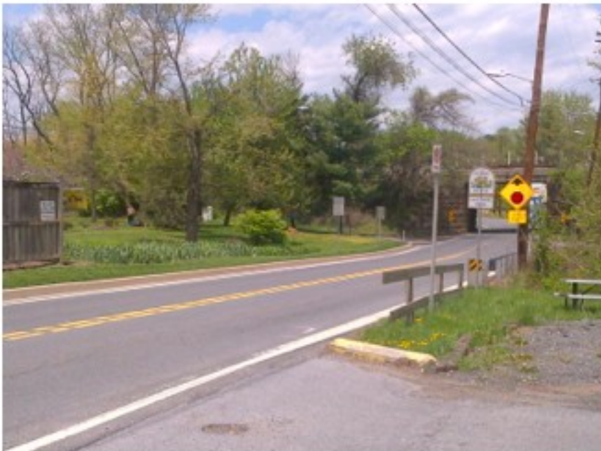
A PLETHORA OF SIGNS AS YOU APPROACH THE RAILROAD UNDERPASS ON RT 28 IN RURAL DICKERSON, MARYLAND
