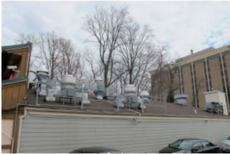
MORE ROOF DETAILS ON A LOCAL CHINESE RESTAURANT
