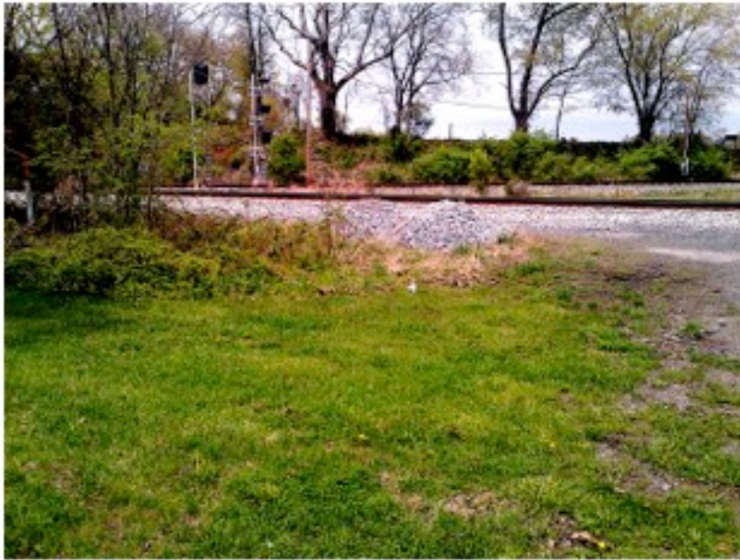
A WYE JUST SOUTH OF FREDERICK, MD. NOTE THE TWO SIGNALS AND BALLAST PILES
